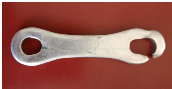
Fig. 8: Fractured 6 mm thick link
